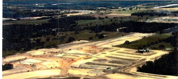
Kelly Park Road Construction, December 2025 Image: WESH 2
